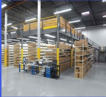
Warehouse Bulk Storage System
